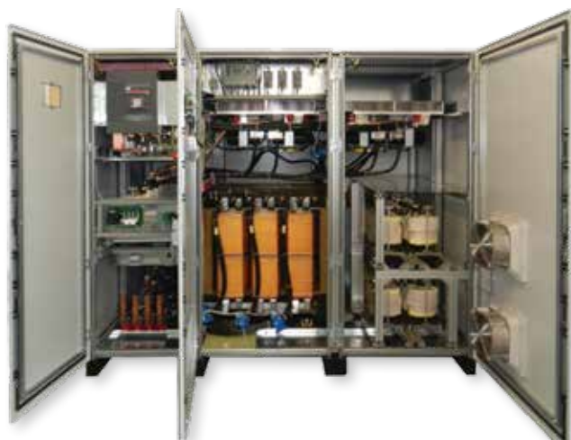
Example of an opened 250kVA FVCT2k Unit
